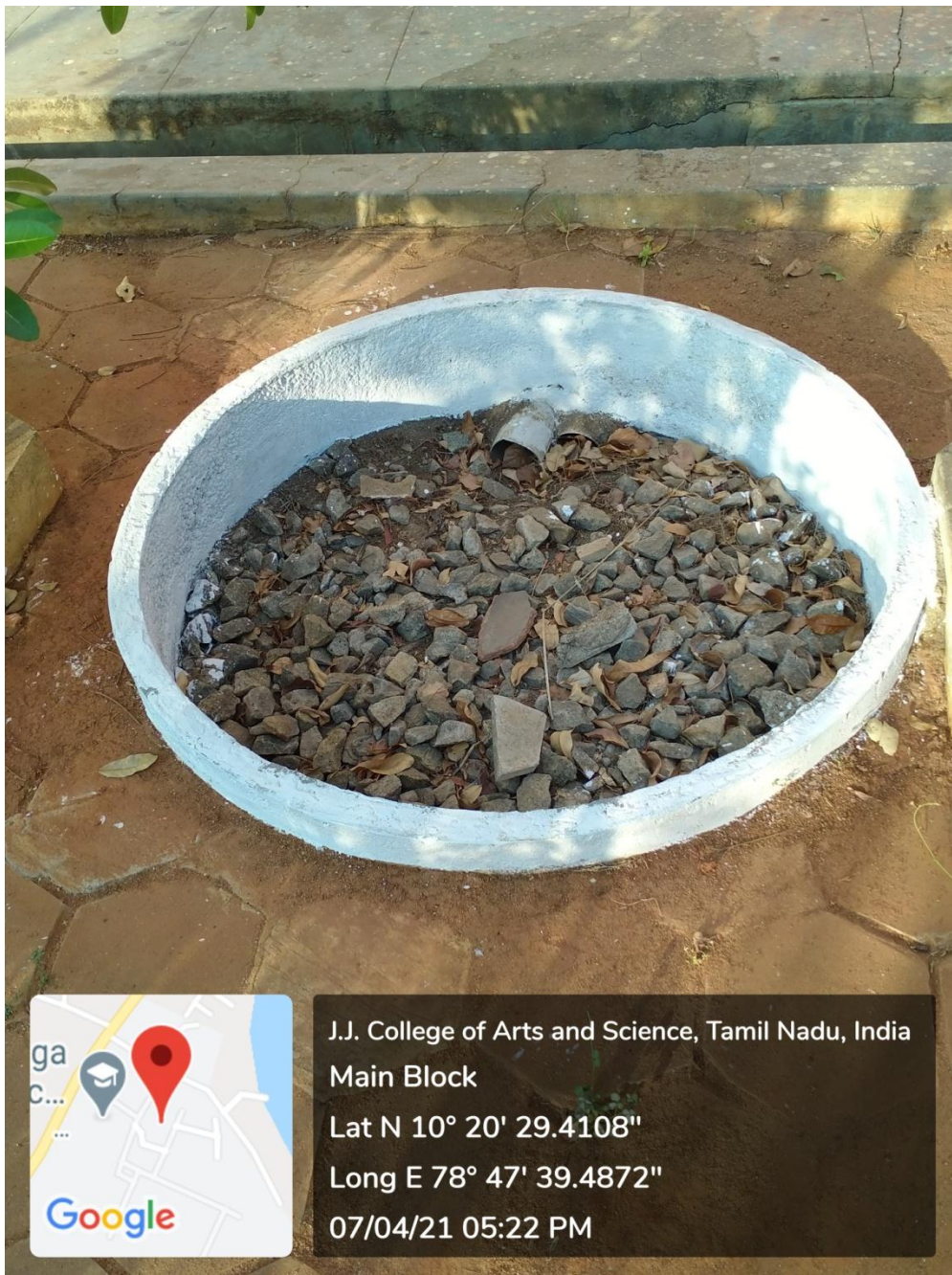
RAIN WATER HARVEST( MAIN BLOCK)
